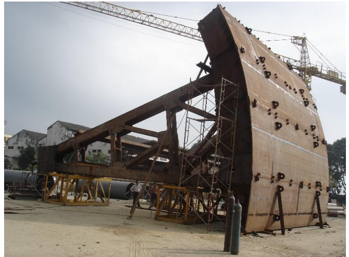
Construction of hydropower valve
