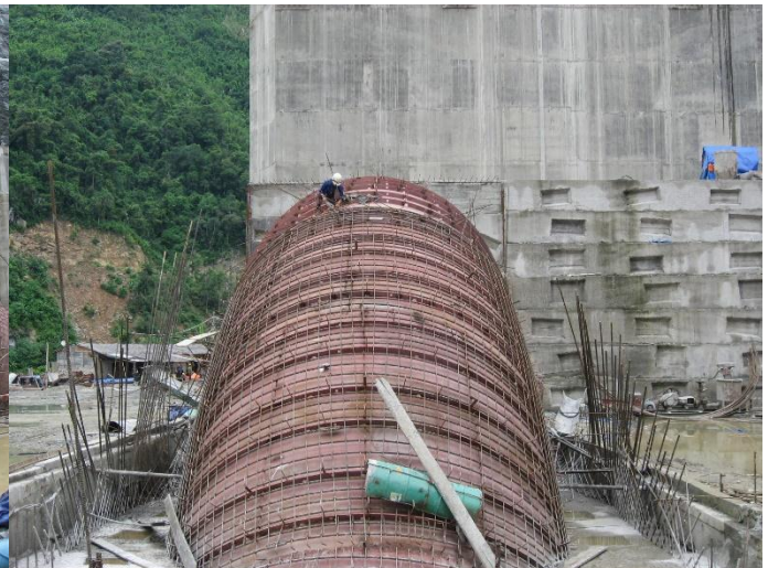
Construction of pressure pipe –Ban Ve hydropower plant
