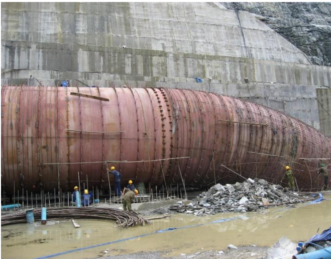
Construction of pressure pipe –Ban Ve hydropower plant
