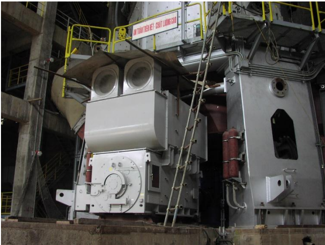
Construction of raw material grinding machine for Bim Son Cement 3
